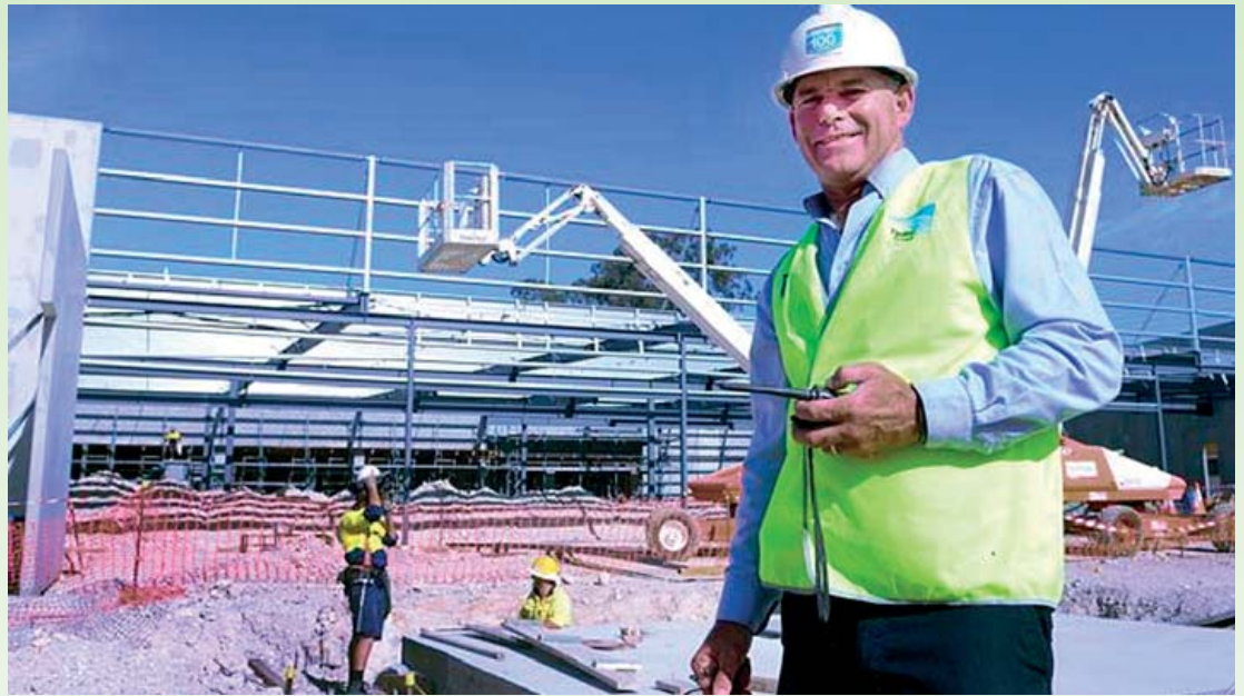
Hutchies' site foreman David Wallace monitors progress at Pimpama Junction.
