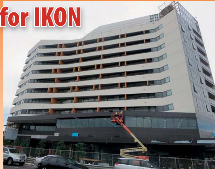
Finishing touches to IKON are now complete.
